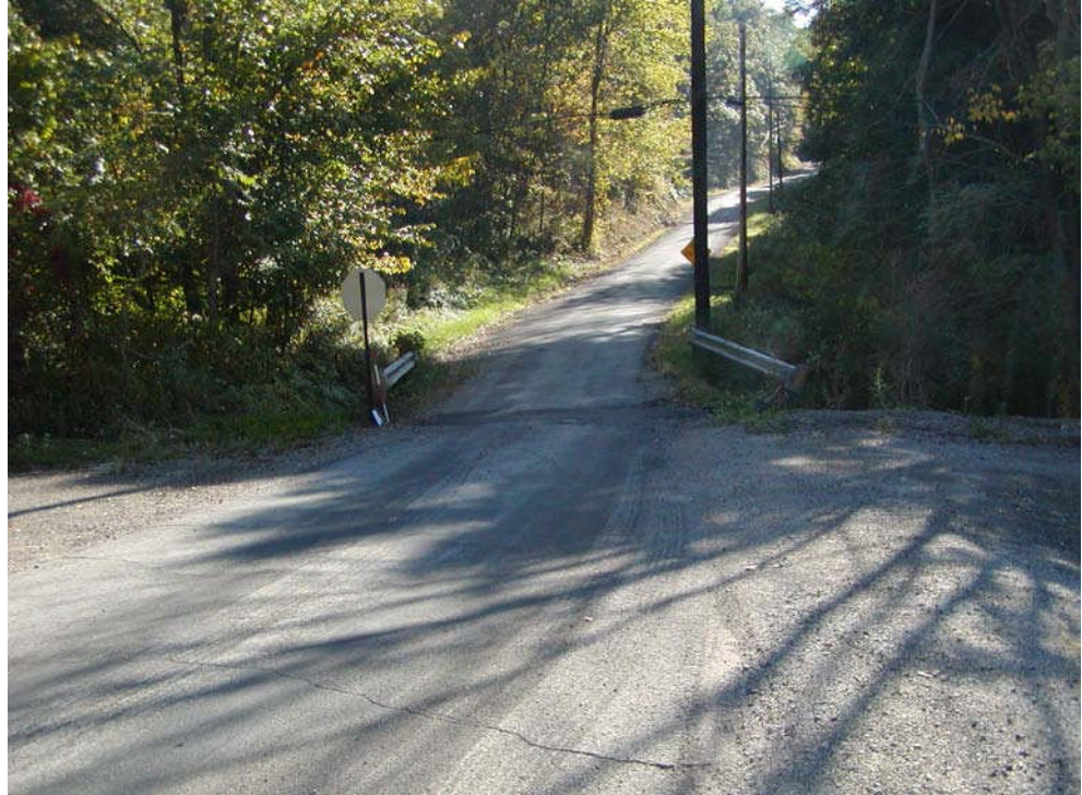
Figure 4.6.1 Near Approach - Toward Bridge
