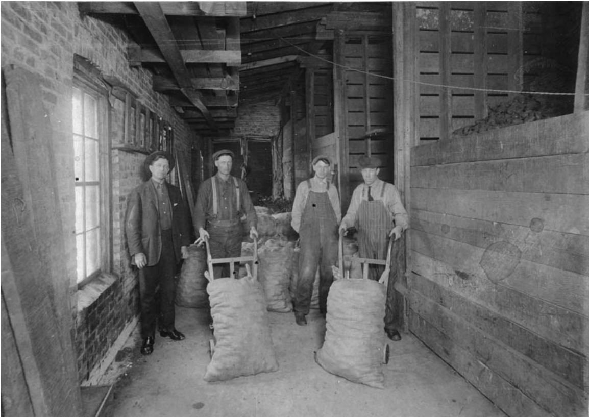
Potato warehouses had large bins in which to store the crop, and slatted bin walls and floors for ventilation. The potatoes were usually stored in a fully- or partially-excavated lower level. The warehouse in this photo is atypically large; it may be on a large farm or be the warehouse of a buyer or middleman. Location unknown, circa 1910. (MHS photo)
