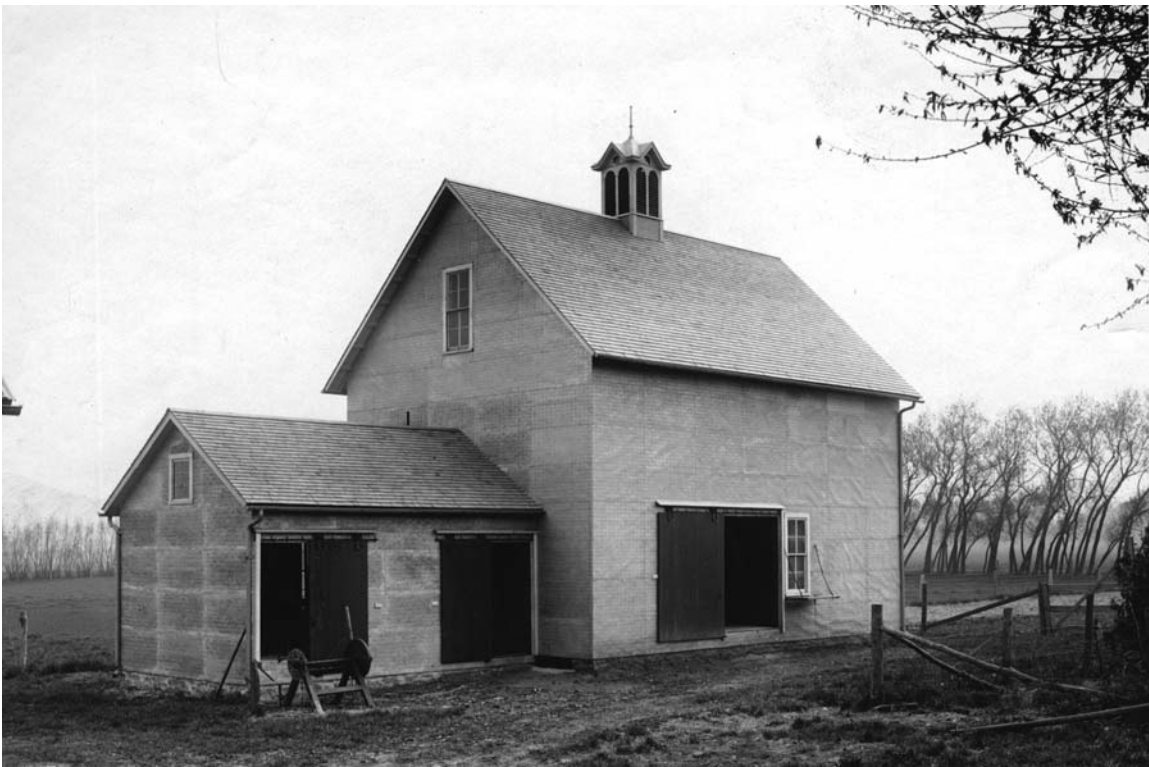
A power house (left), grinding tool (front), and granary (right). Both buildings were covered with pressed metal siding simulating brickwork. Location unknown, circa 1910. (MHS photo by Harry Darius Ayer)
