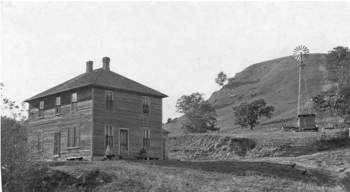
A pump house at the base of a windmill. Photograph taken near Welch in Dakota County, circa 1909. (MHS photo)
