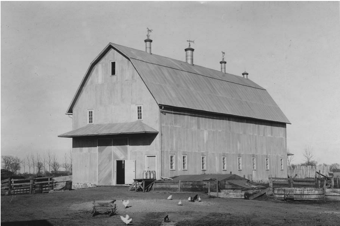
Most dairy barns had passive gravity ventilation systems with outlet flues topped with metal caps and/or wooden cupolas. The fresh air intakes were usually along the barn's sidewalls. This barn was covered with sheets of corrugated metal, a low-maintenance material that was in use by the early 20th century. Six milk cans stand near the door in this photo. Location unknown, circa 1910. (MHS photo by Harry Darius Ayer)
