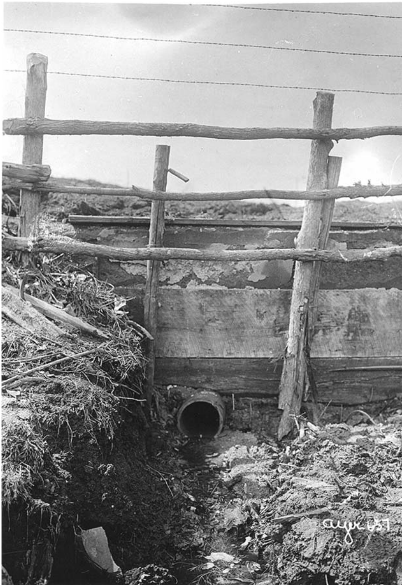
This drain tile required structural support at its outlet to the ditch. Location unknown, circa 1910. (MHS photo by Harry Darius Ayer)
