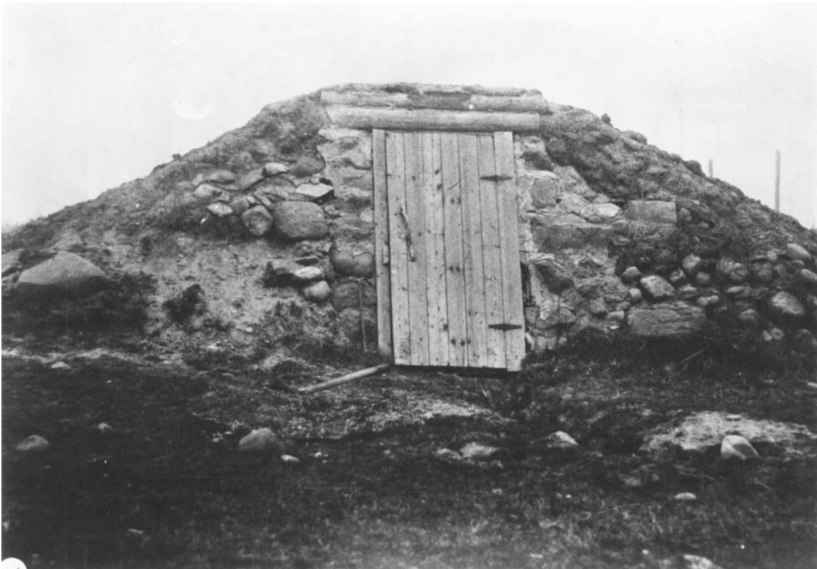
Many root cellars were built of stone rubble. Some were dug into hillsides; others were partly excavated and then banked with earth and sod. Konristo Farm, Carlton County, 1918. (MHS photo by St. Paul Dispatch )
