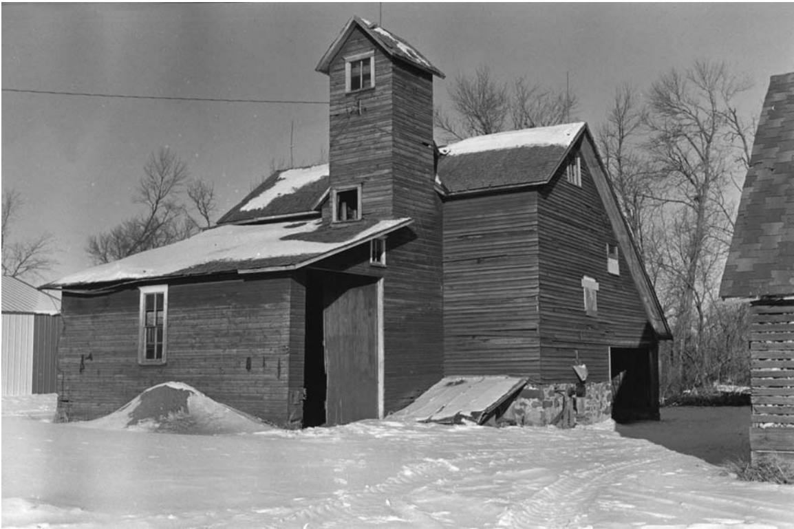
Built circa 1885, this farm elevator had woodframe construction, clapboard siding, a scale for weighing, and elevating equipment that filled at least seven overhead bins. The elevator was also used for machinery storage. Twente Farm, Brown County, 1979. (MHS photo by Gimmetstad)
