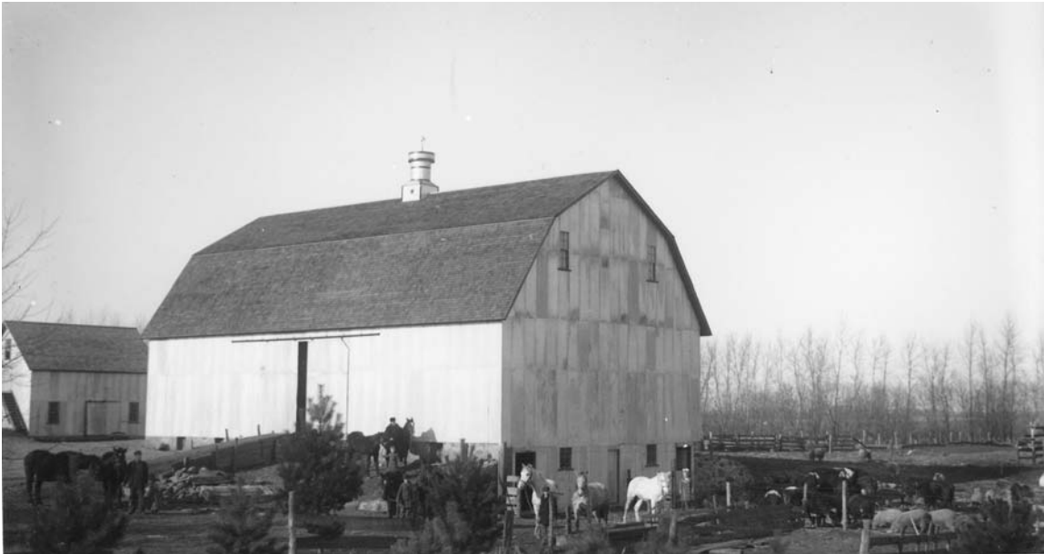
This barn was covered with corrugated metal panels. There are horses, cows, sheep, and hogs in the adjacent yards. Trygeseth Farm, Yellow Medicine County, circa 1915. (MHS photo by Ole Mattiason Aarseth)
