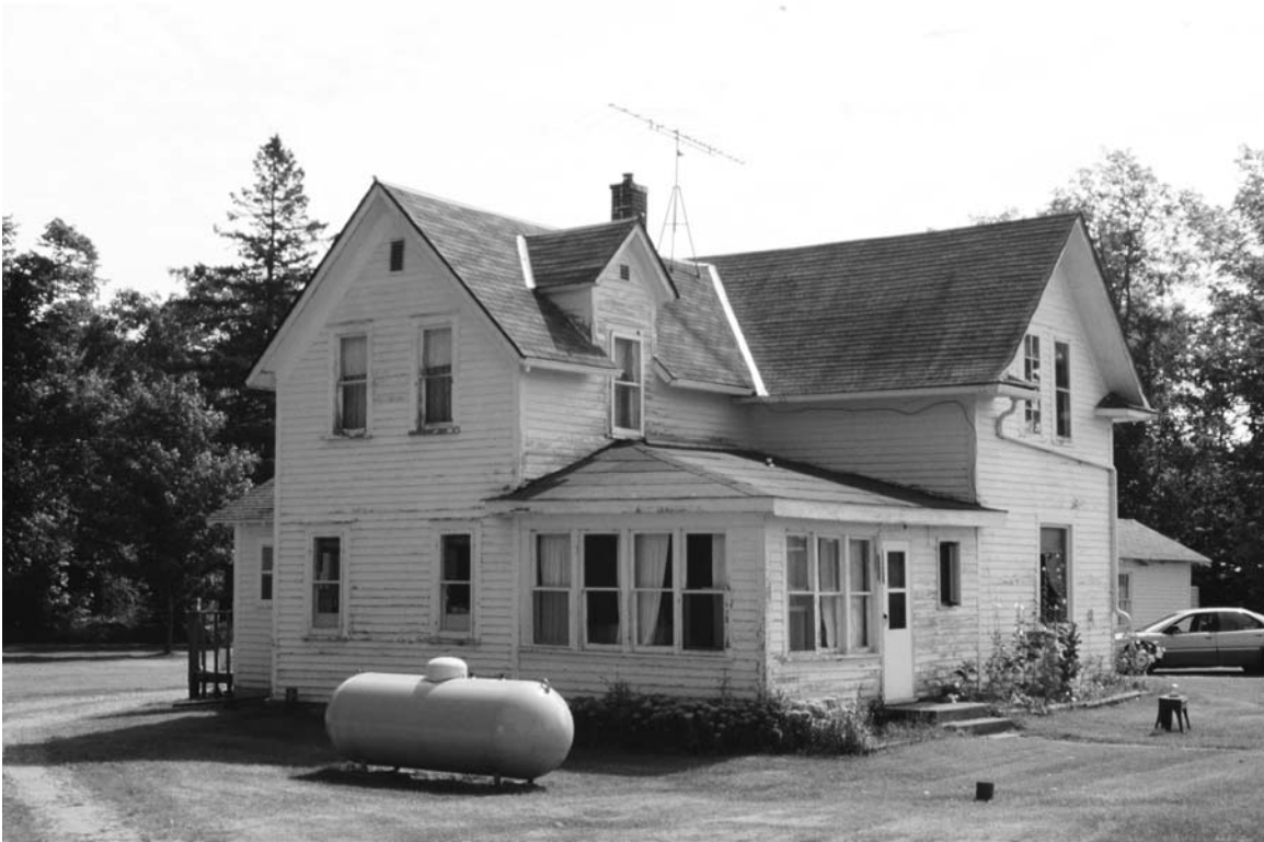
Bulk propane tanks usually stood near the farmhouse, or between the farmhouse and another building in which the fuel was needed. Propane was commonly used for heating and cooking, as well as for drying crops, fueling brooders, etc. Scott Farm, Garrison Township, Crow Wing County, 2003. (Gemini Research photo)
