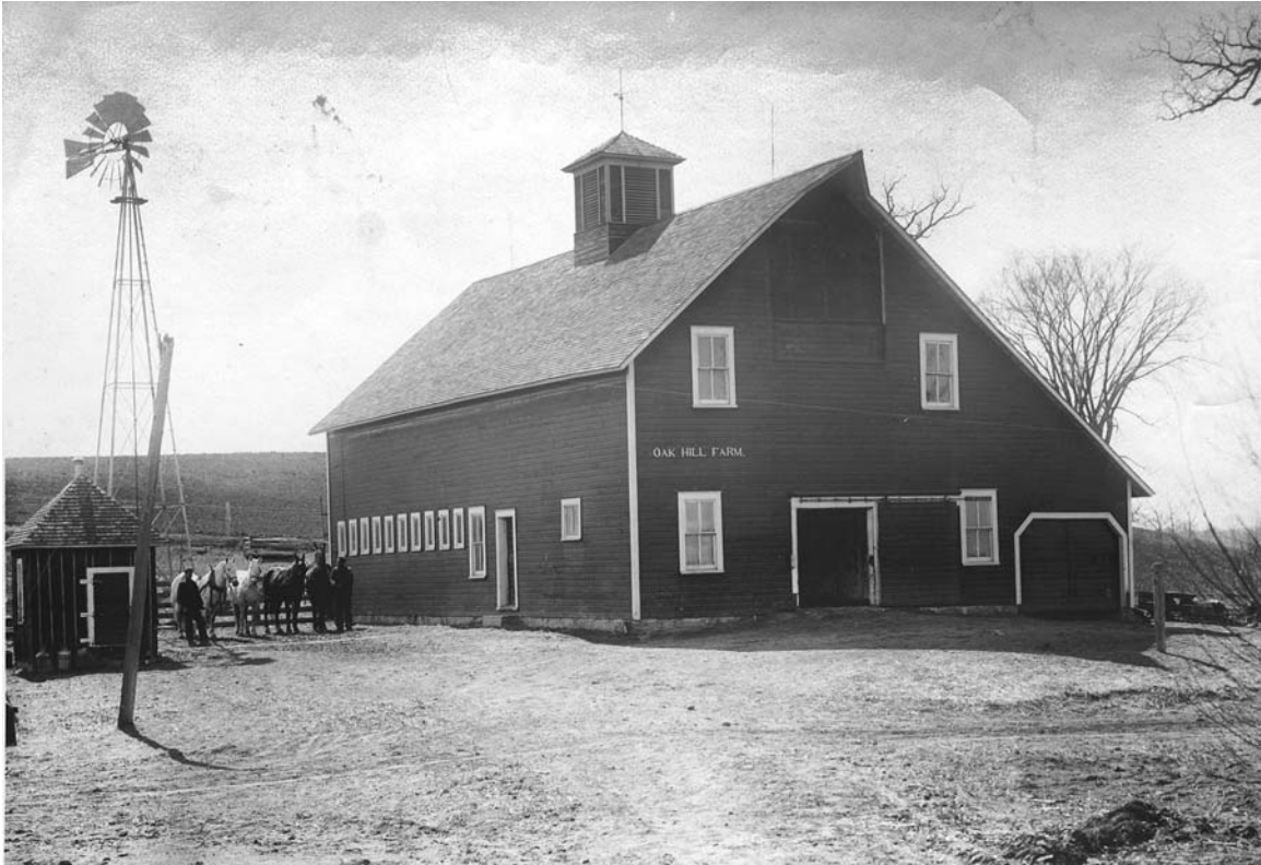
This general purpose or combination barn housed horses and cattle. Note the closely spaced windows, one for each stall. Oak Hill Farm, location unknown, circa 1910. (MHS photo by Harry Darius Ayer)
