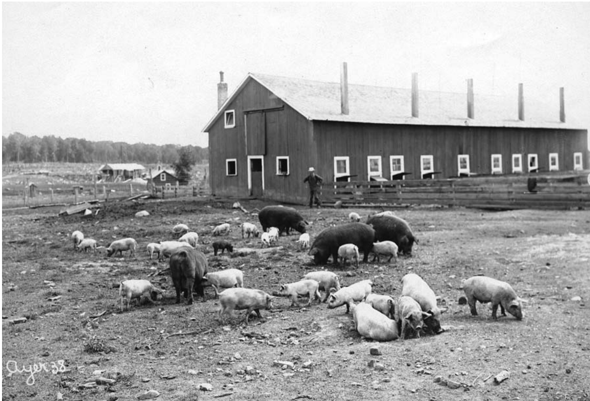
Sows with their litters in a hog yard. This hog barn had an upper loft for bedding and a ventilation system with flues for each pen. This barn's flues were tall to help them draw correctly. Note the sturdy board fence. Location unknown, circa 1910. (MHS photo by Harry Darius Ayer)
