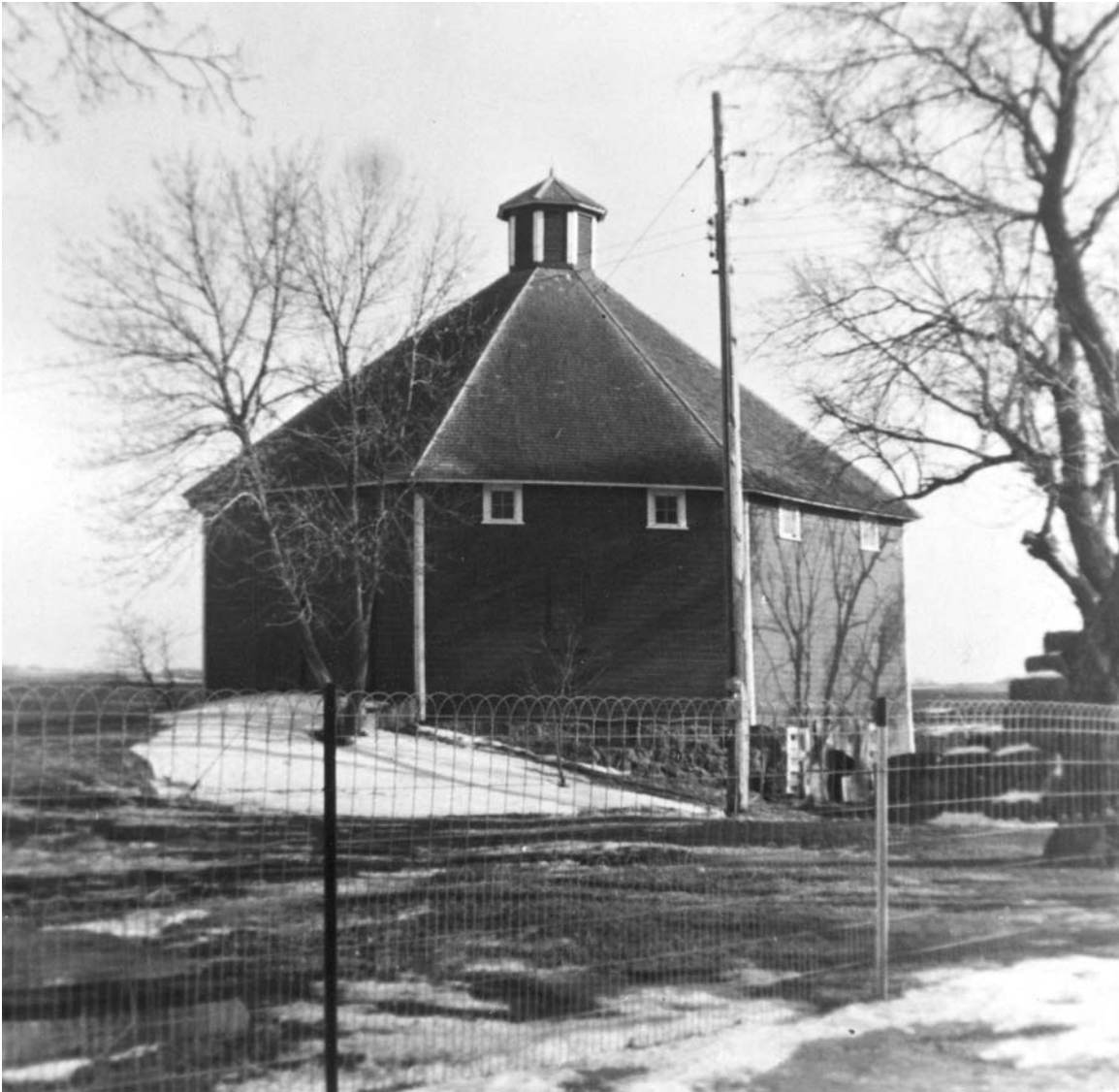
One of many styles of woven wire fence that were commercially available. This fence had steel posts, which were common on Minnesota farms by the 1930s. Miller Farm, Lac qui Parle County, circa 1950. (MHS photo)
