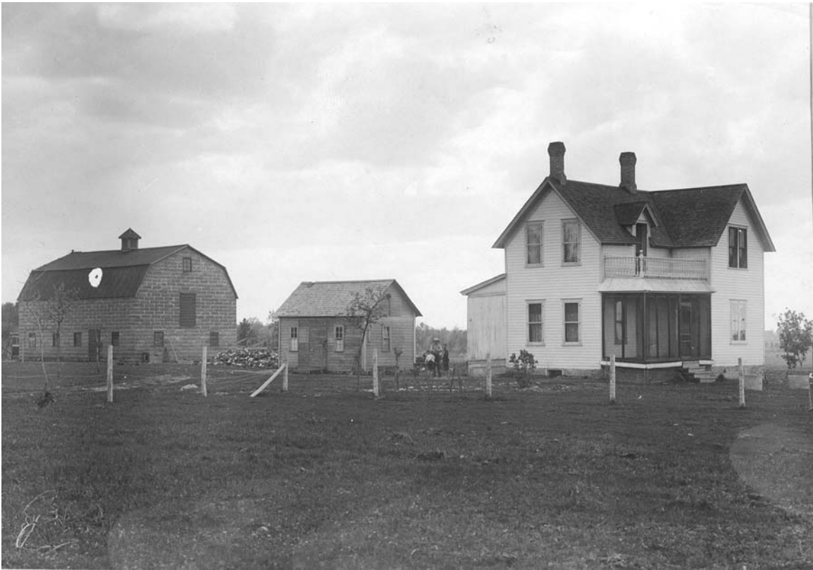
After a larger farmhouse was built, the earlier, smaller house was commonly reused as a summer kitchen, bunkhouse, granary, shop, or shed. In this photo, the earlier house stands behind its replacement. Crow Wing County, circa 1910. (MHS photo by Harry Darius Ayer)
