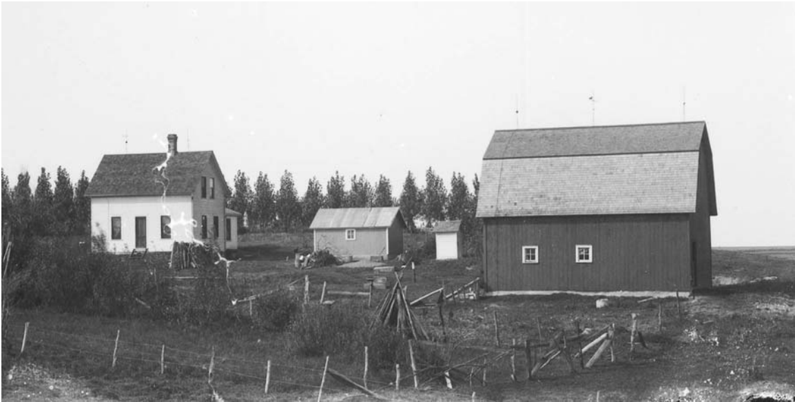
This moderately-sized general purpose barn had vertical siding and three lightening rods on the roof. Location unknown, circa 1900. (MHS photo by John T. Austinson)
