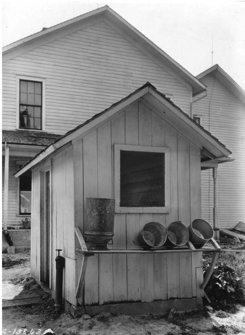
An adequate milk house could be as small as 8' x 8', although a 10' x 12' design was more accommodating. This house had a concrete foundation, wood siding, and an outside drying rack, all typical. The black device (with handle) near the door was probably an insulated water shut-off valve. Believed to be Douglas County, circa 1950. (MHS photo)
