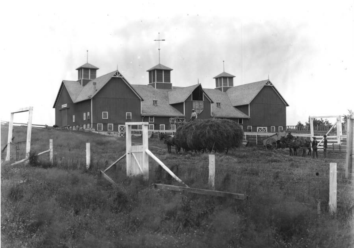
Two whitewashed wooden gates marked openings in a woven wire fence that had round wooden posts. One gate was the width of a wagon and the other was more narrow. Many farmers preferred woven wire fences because they held sheep and hogs, which barbed wire couldn't contain, and because they didn't have sharp barbs that injured valuable horses and dairy cows. Location unknown, 1914. (MHS photo by Charles J. Hibbard)
