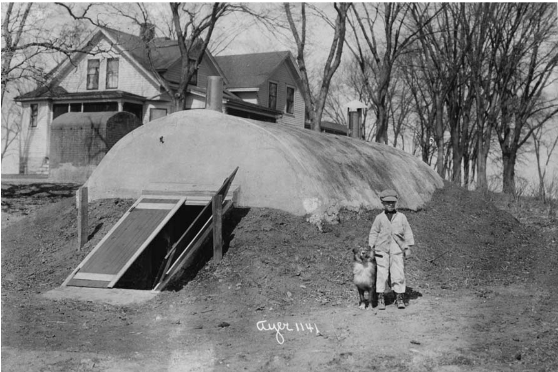
This ground cellar may have been built of canvas stretched over curved sticks and rough boards. Note the ventilation flues. Location unknown, circa 1910. (MHS photo)
