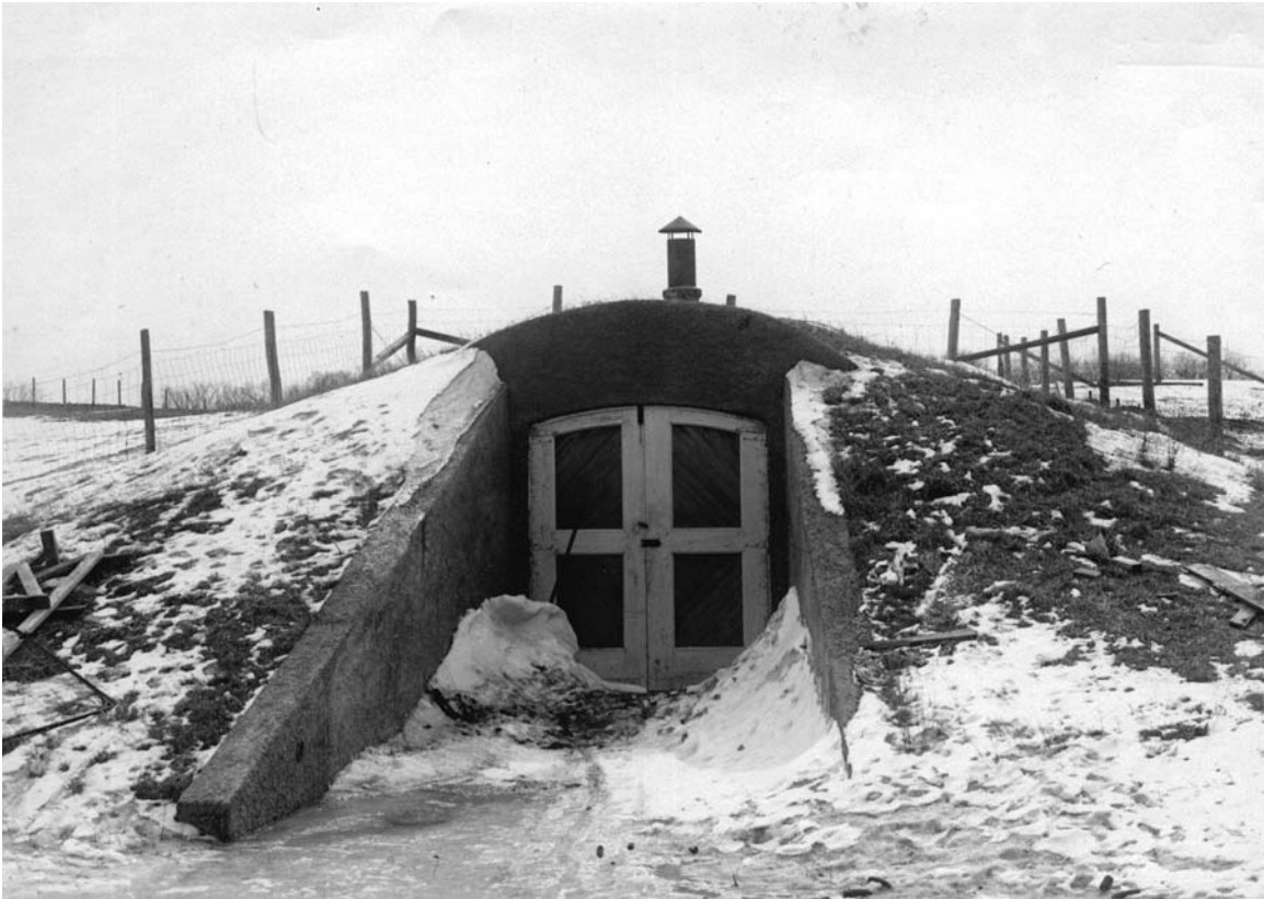
A ground cellar of at least part concrete construction, covered with sod and ventilated. Location unknown, circa 1910. (MHS photo)
