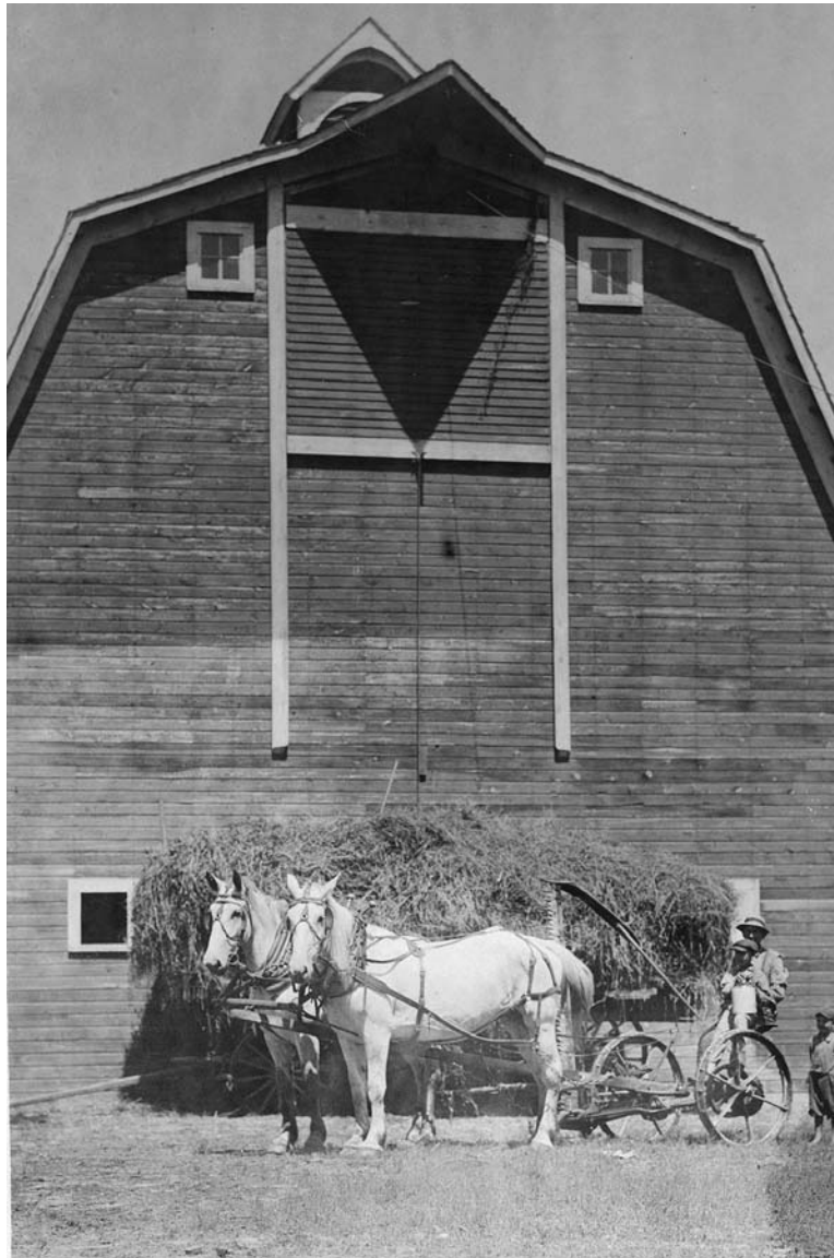
A load of hay ready for the loft. One Minnesota farmer in 1914 advised that the hay door be placed on the northern end of the barn so that the hot dusty chore of loading the hay in August could be done in the shade (Henry 1914). While second story lofts saved labor at feeding time, the dry hay was highly flammable and barn fires were common. Location unknown, circa 1910. (MHS photo by Harry Darius Ayer)
