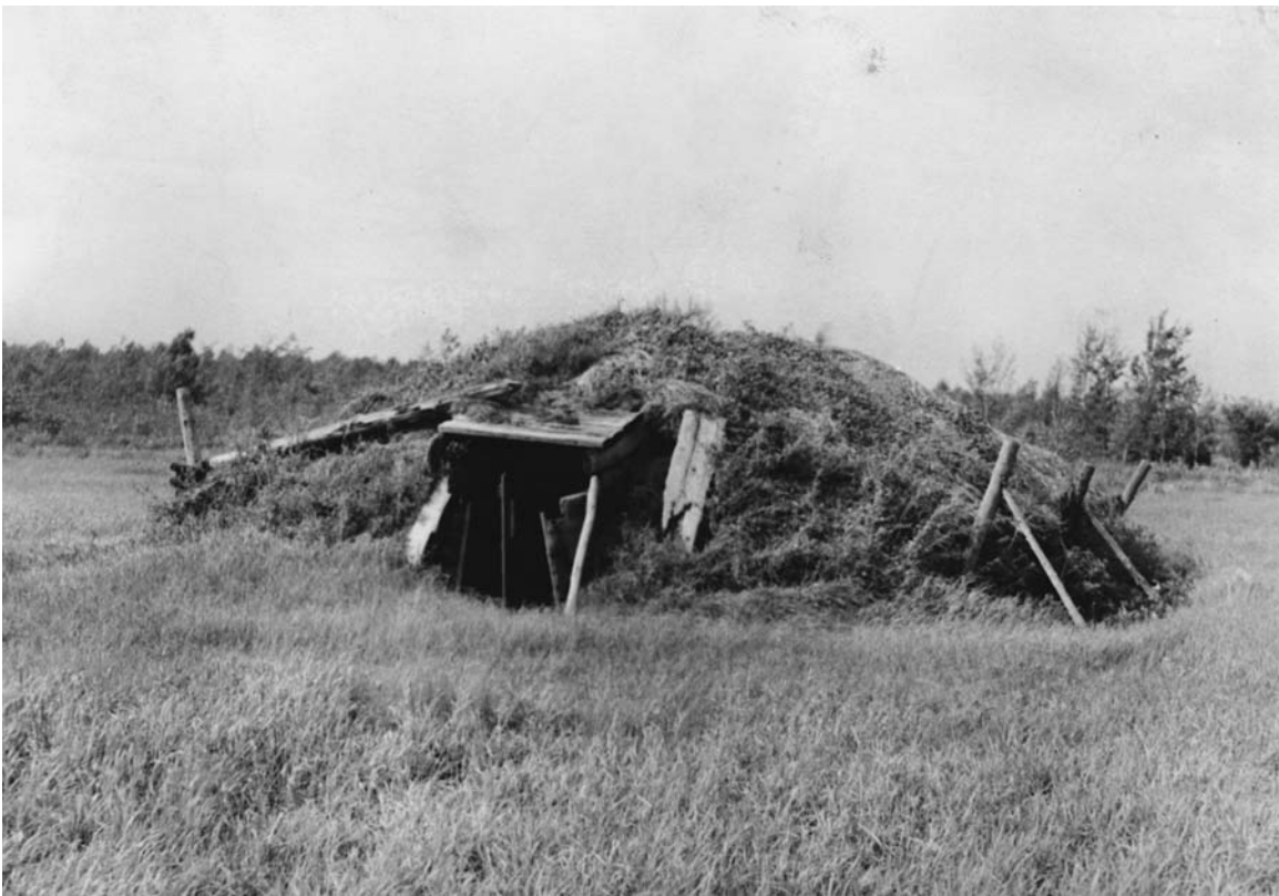
Root cellar (a ground cellar type) of Finnish construction. John Kurnicki Farm, St. Louis County, 1937. (MHS photo)
