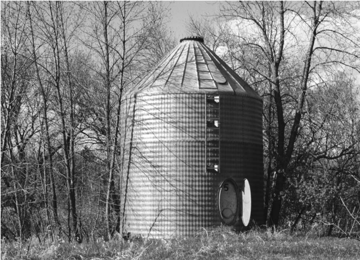
A metal grain bin located near the edge of a field, rather than within the farmstead. It has two hinged, oval hatch doors – a small door on the roof for filling and a larger door near the base for unloading. Framnas Township, Stevens County, 2004. (Gemini Research photo)
