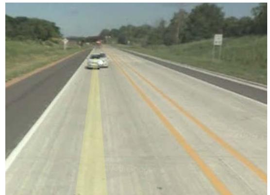
Figure 30 - Four-foot buffer with rumble strips
