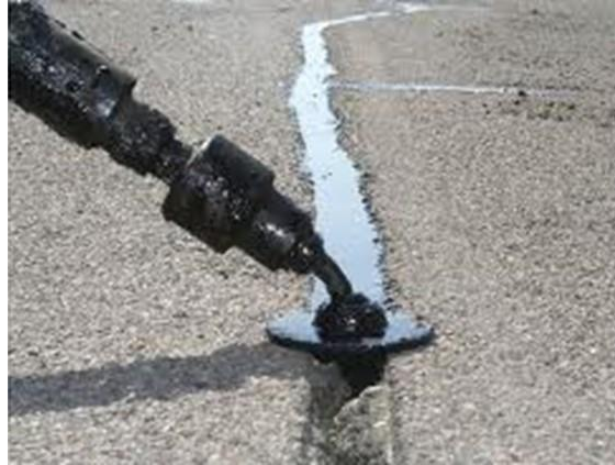
Figure 100.11 – Crack sealant applied from the wand.
