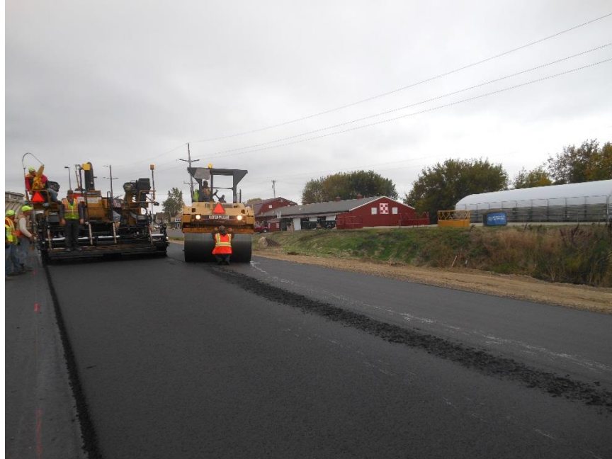
Figure 600.26 – Steel drum roller picking up mix.
