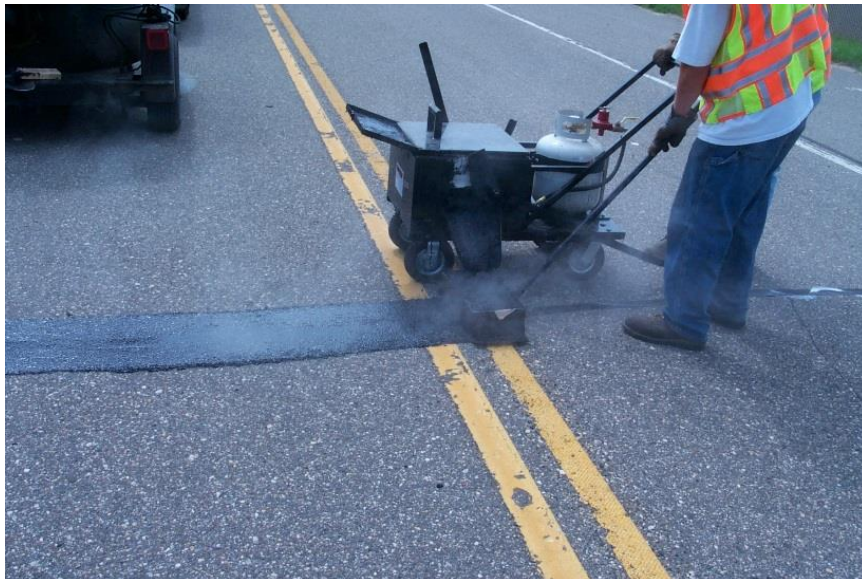
Figure 100.13 – Mastic being applied to a cupped transverse crack.
