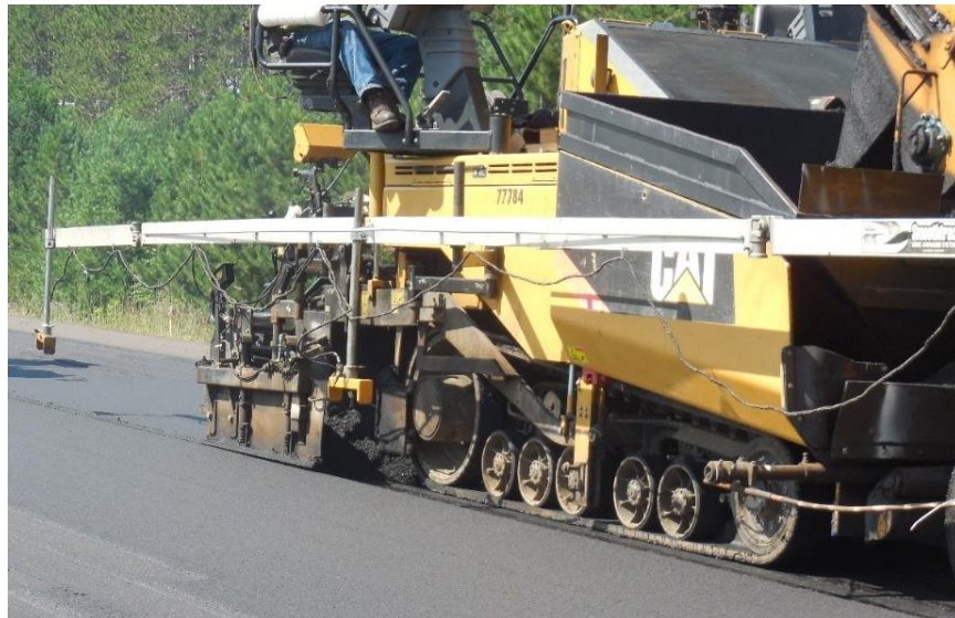
Figure 500.16 – A tracked paver using sonics to adjust the screed.
