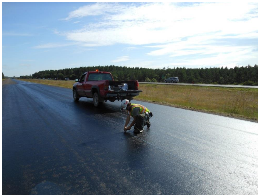
Figure 600.31 – Contractor setting stringline to guide the paver
