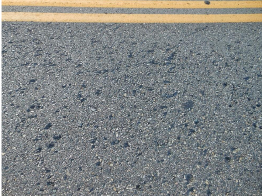
Figure 600.17 – The result of excessive spall material in a mix. This may have a profound effect on the long-term durability of the pavement.
