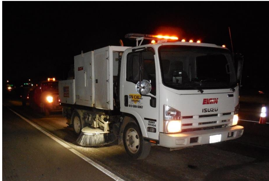
Figure 500.4 – Broom truck preparing the existing surface for overlay.
