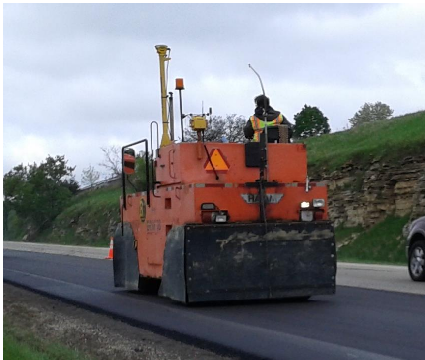
Figure 600.27 – Pneumatic-tired roller with skirt to retain wheel heat
