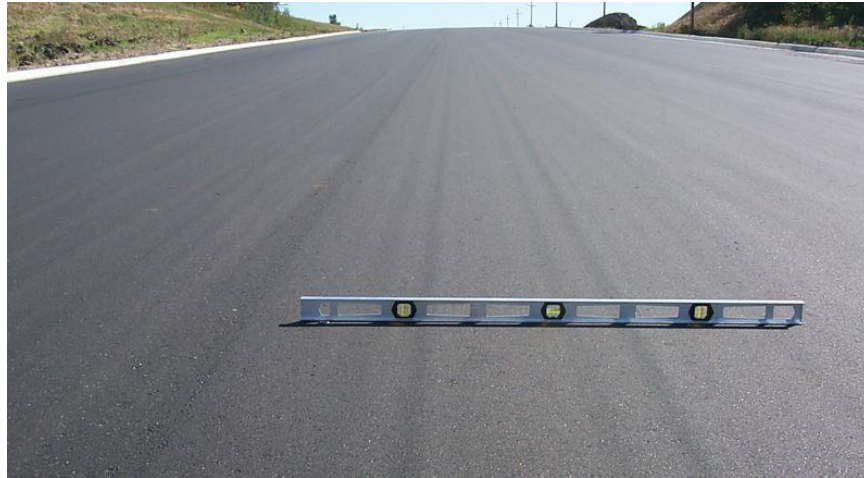
Figure 600.24 – Roller marks
