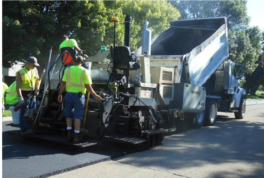
Figure 500.7 – An end-dump truck delivers bituminous mix directly into the paver hopper.
