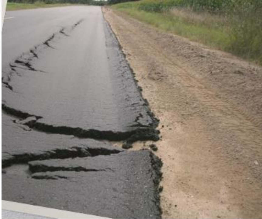
Figure 600.23 – Yielding of the aggregate base
