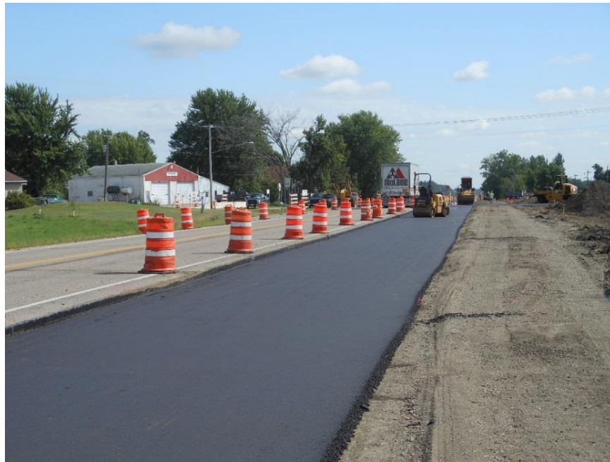
Figure 500.1 – Paving operation within a traffic control setup.
