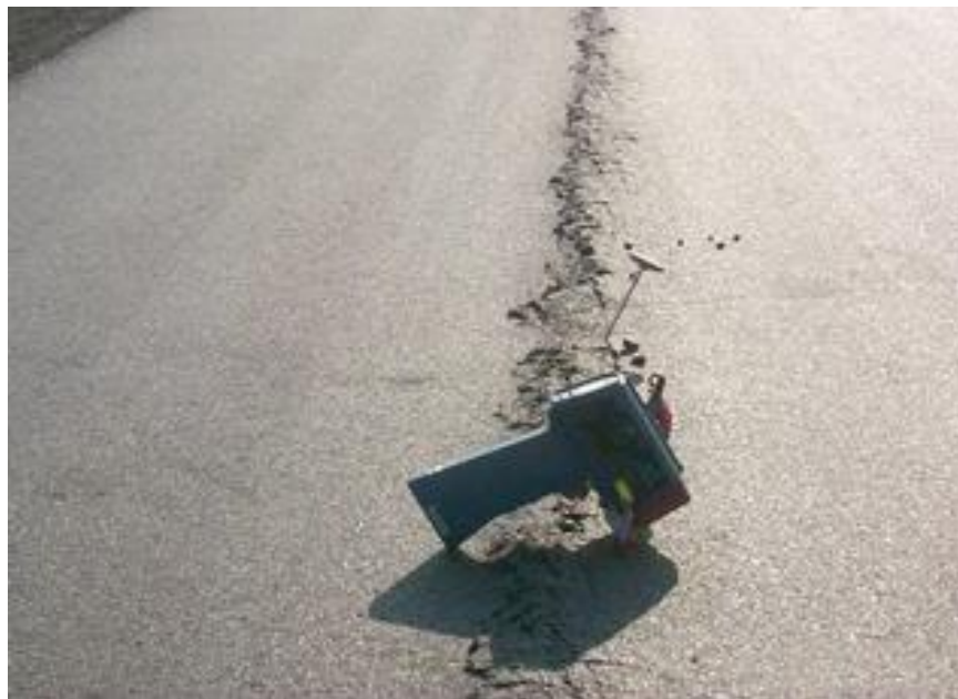
Figure 600.15 – Tearing of the mat in the tender zone
