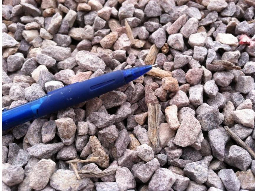
Figure 200.18 – Aggregate mix contaminated with pieces of wood, which is considered deleterious material.
