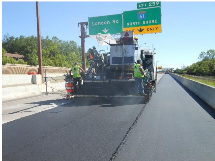
Figure 100.3 – Ultrathin Bonded Wearing Course
