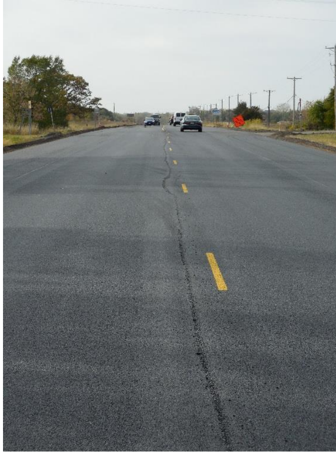
Figure 600.30 – Wavy Longitudinal Joint
