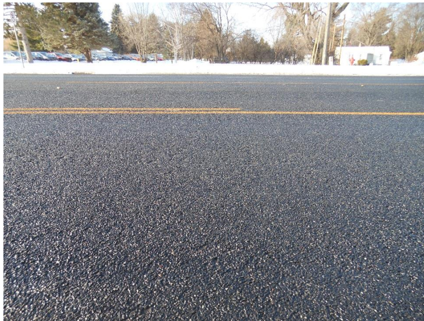
Figure 100.7 – Bituminous Seal Coat.
