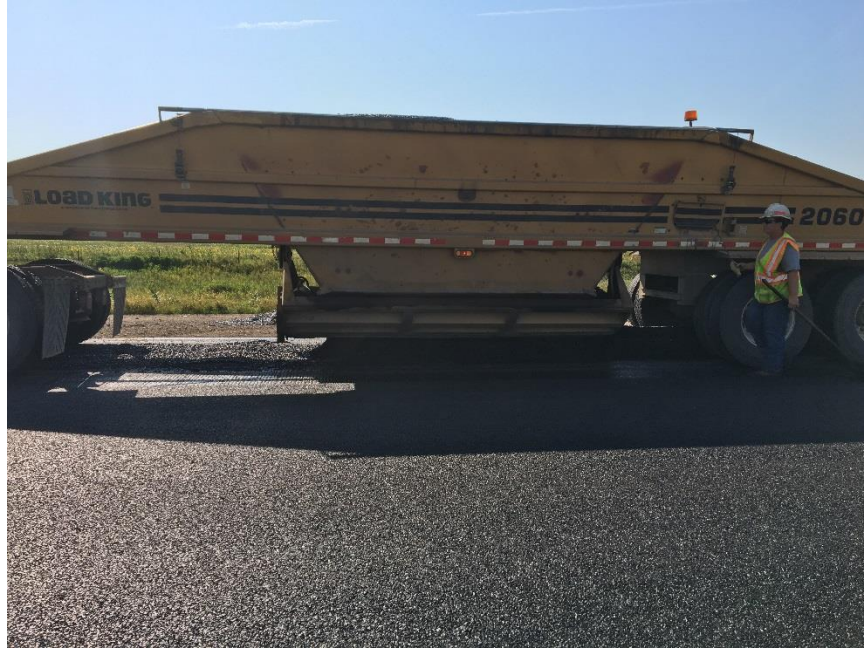
Figure 500.8 – A belly-dump truck windrowing a load of asphalt.
