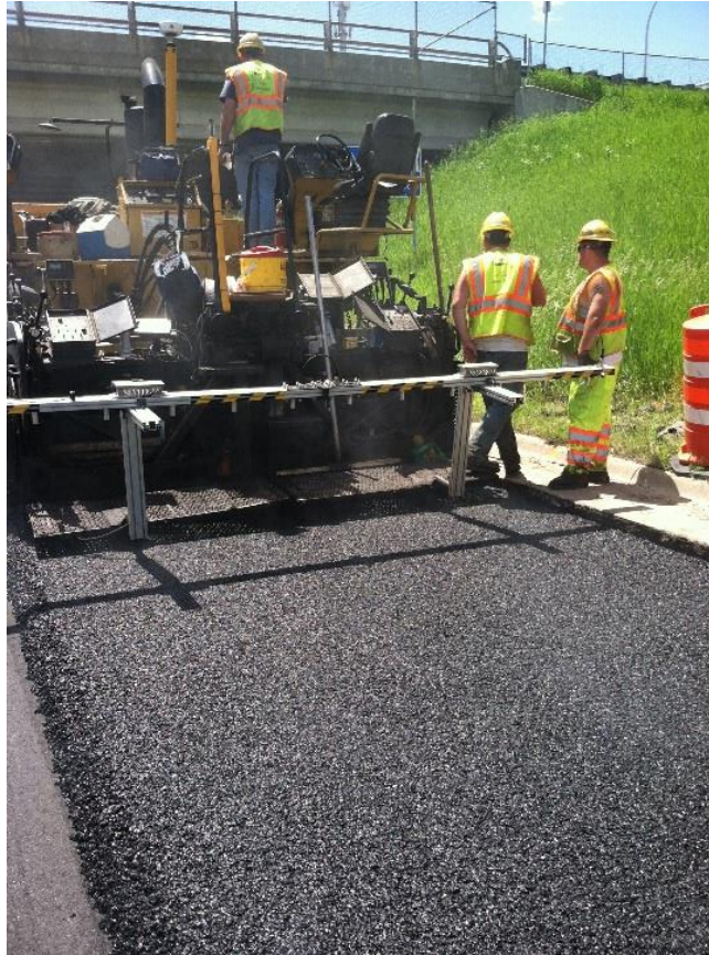
Figure 100.5 – SMA being placed over a bituminous surface.
