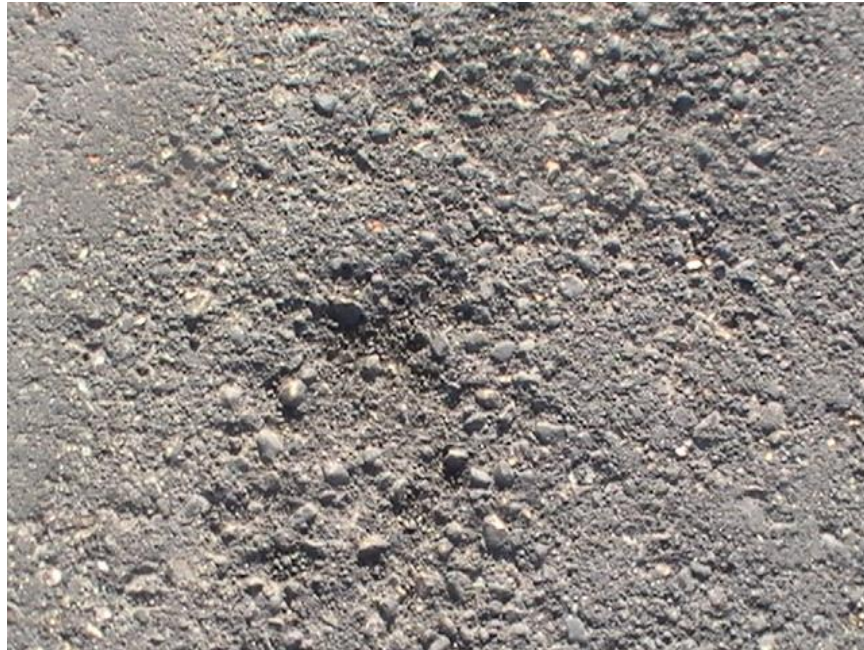
Figure 100.19 – Raveled pavement.
