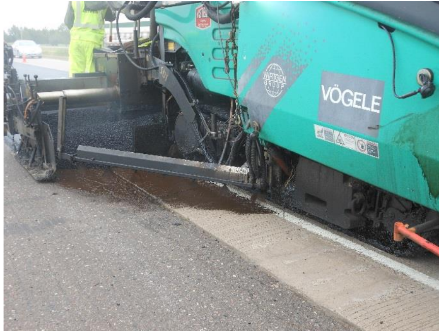
Figure 100.2 – Spray paver applying tack and UTBWC
