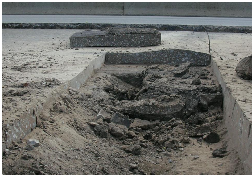
Figure 600.29 – Analysis of a bump over a concrete joint. Note that the bump actually forms a bit downstream of the existing concrete joint.
