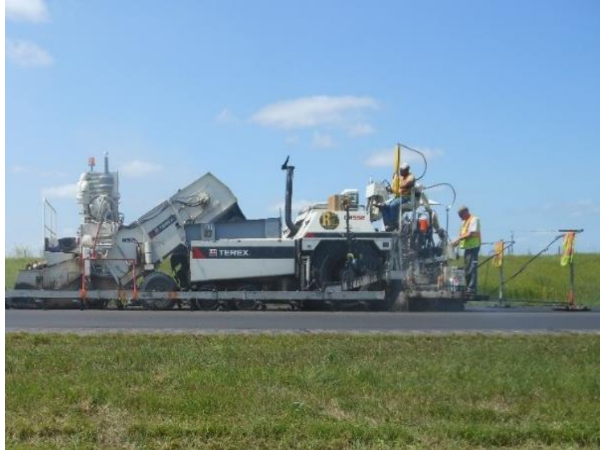
Figure 500.15 – A wheeled paver with contact sensors and pickup machine
