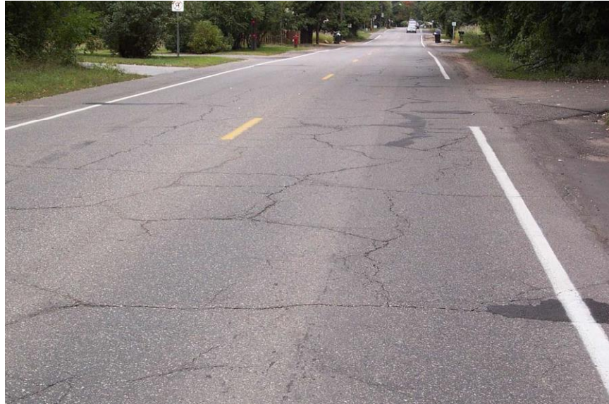
Figure 100.16 – Block Cracking
