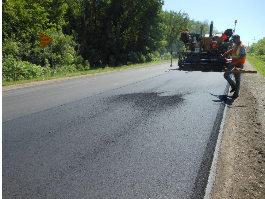
Figure 600.39 – Screed worker broadcasting mix across the mat surface.
