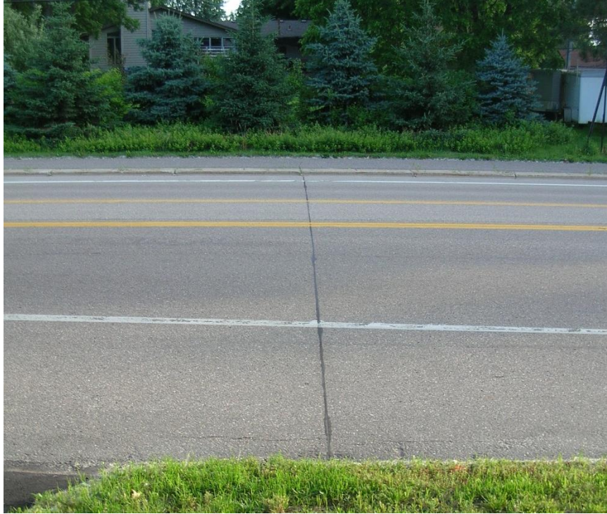
Figure 200.19 - Saw and Seal roadway.
