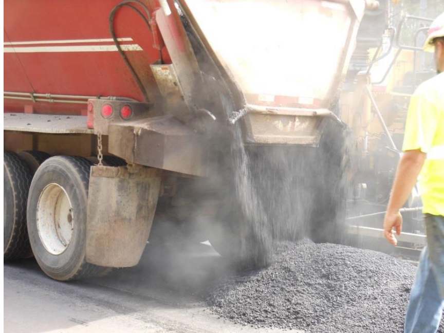
Figure 500.9 – A flow-boy windrows bituminous mix
