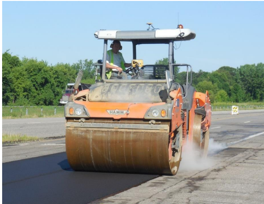
Figure 500.18 – Vibratory Double Steel Drum Breakdown Roller
