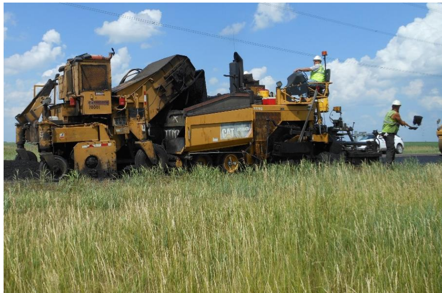
Figure 500.11 – A non-remixing pickup machine transfers bituminous mixture to the hopper.
