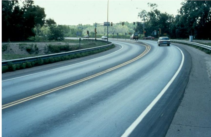
Figure 600.11 – Pavement Flushing
