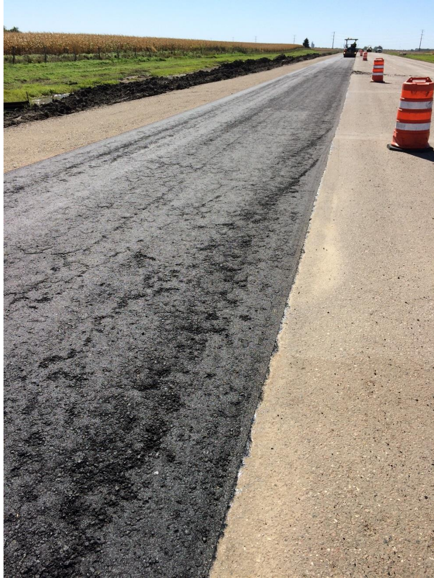
Figure 600.25 – Pneumatic Tired Roller picking up mix.
