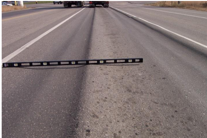
Figure 100.18 – Pavement Rutting
