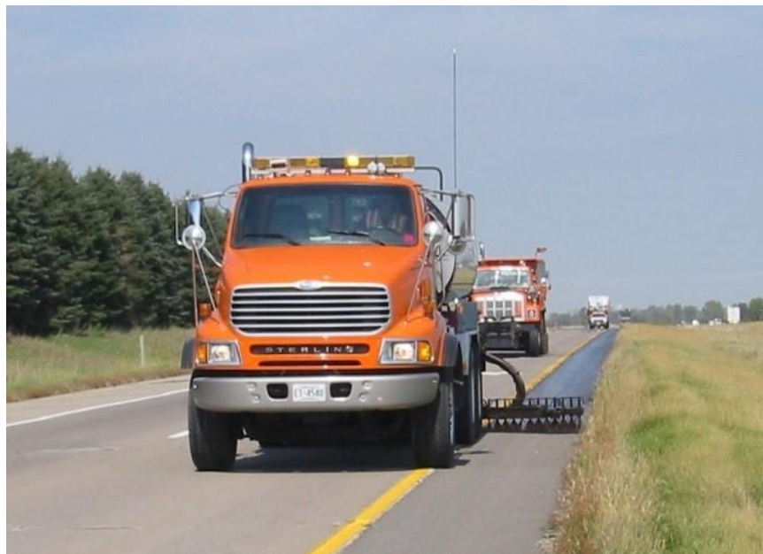
Figure 100.10 – Bituminous Fog Seal being placed on a bituminous shoulder.
