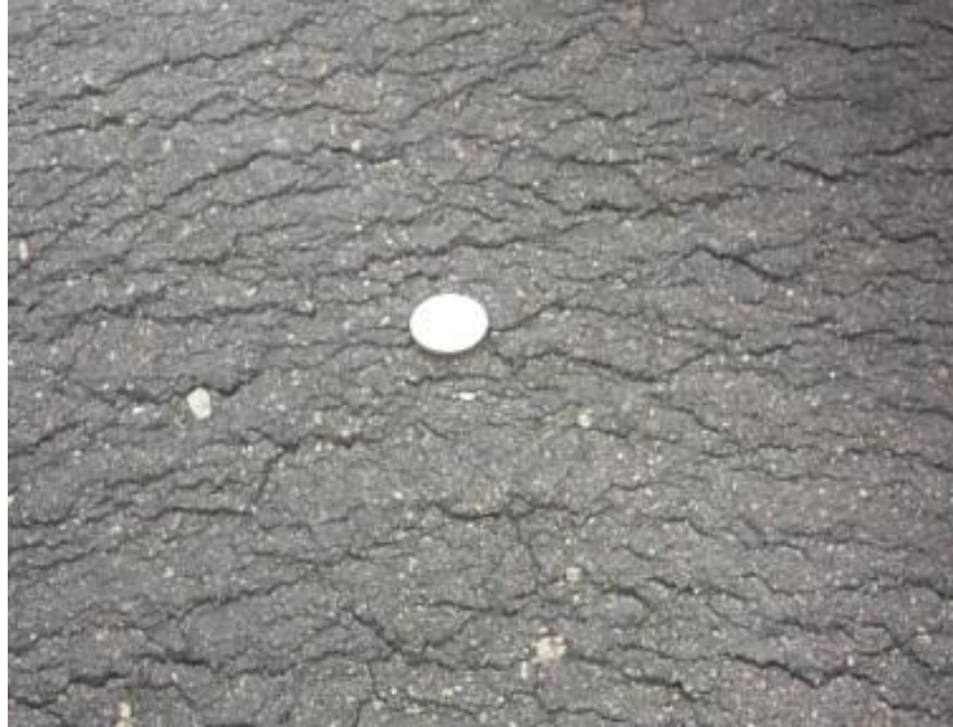
Figure 600.22 – Checking of the mat
