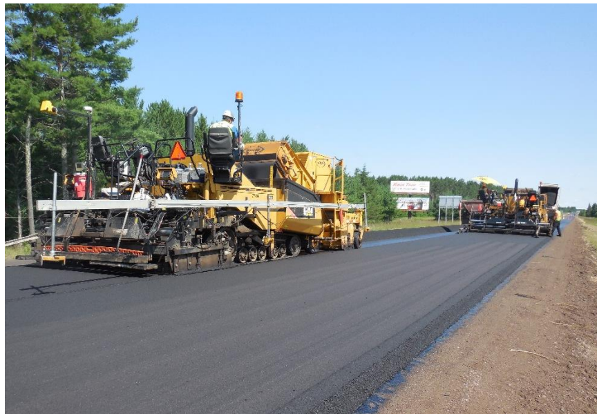
Figure 500.21 – Two pavers in echelon. Two lanes are paved in one operation.
