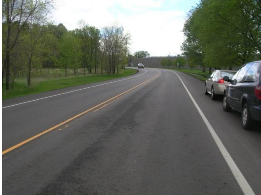
Figure 600.2 – Side to side segregation
