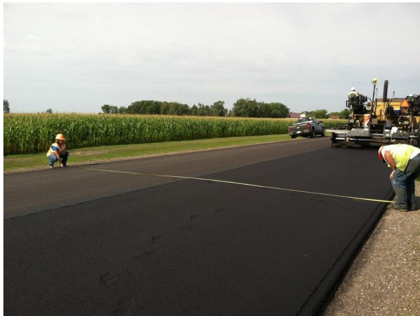
Figure 500.20 – Inspectors measuring the paved width of the road
