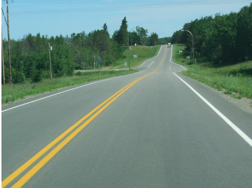
Figure 100.1 – Plant Mixed Asphalt Pavement
