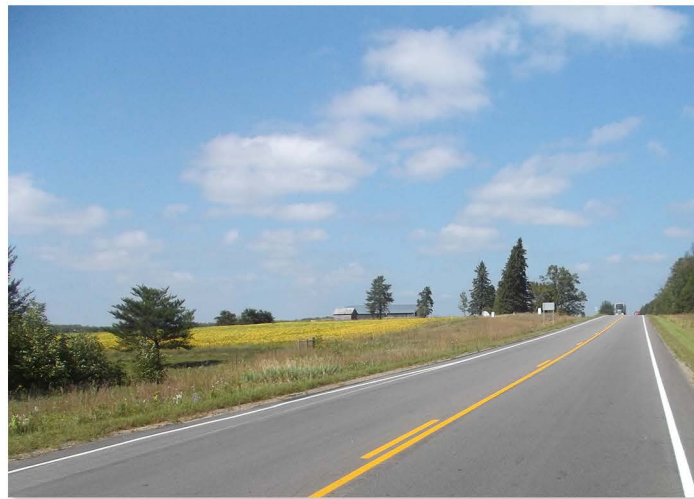
TH64 Condition After 1 Year
