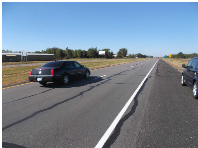
TH23 One Year After Traditional Micro Surfacing
