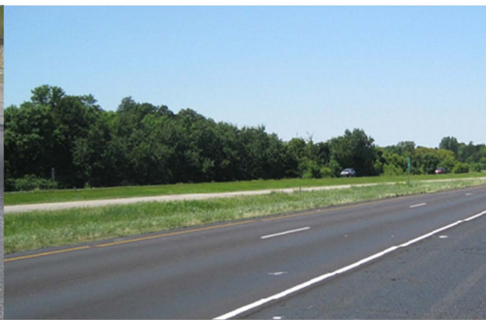
Cell 1 After Micro Surfacing and 1st Winter 2013
