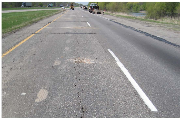
Cell 1 Before Micro Surfacing 2012
