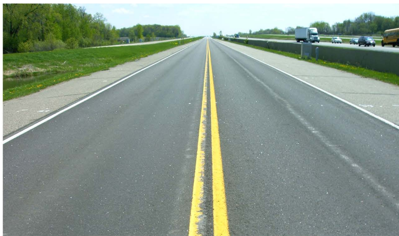
MnROAD Cell 24 - 8 Months After Placement
