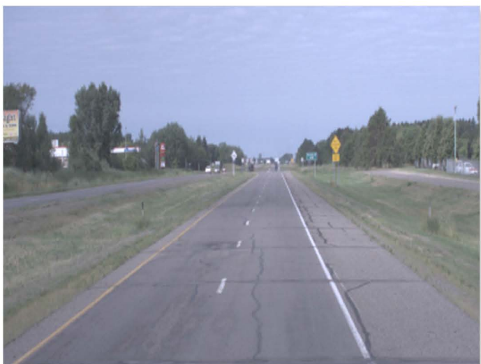
TH23 Before Traditional Micro Surfacing
