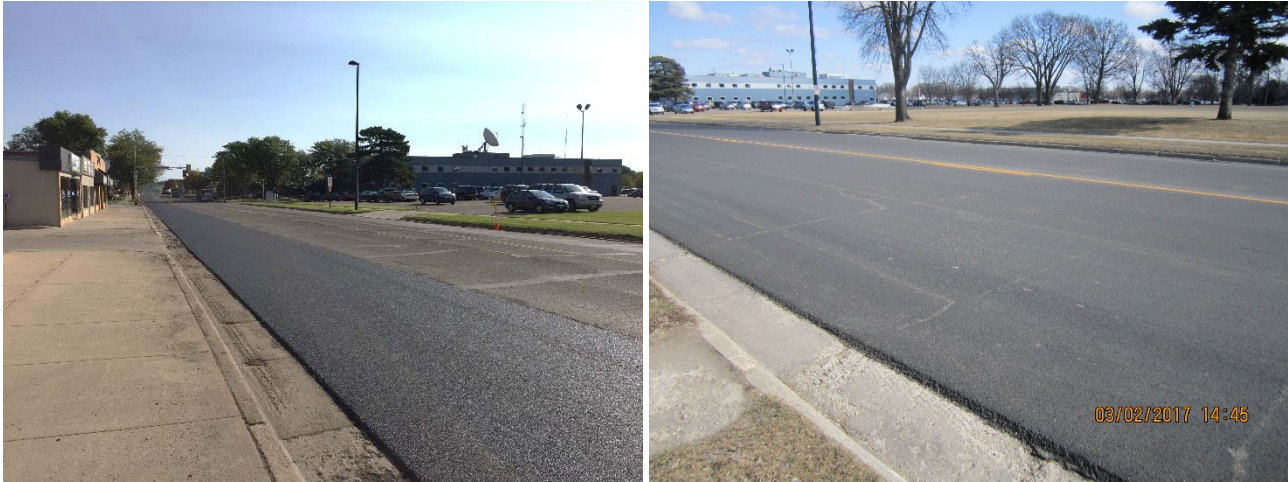
Figure 5 Minnesota Trunk Highway 15: (Left) during 2016 UTBWC mill and overaly, (Right) spring 2017.
