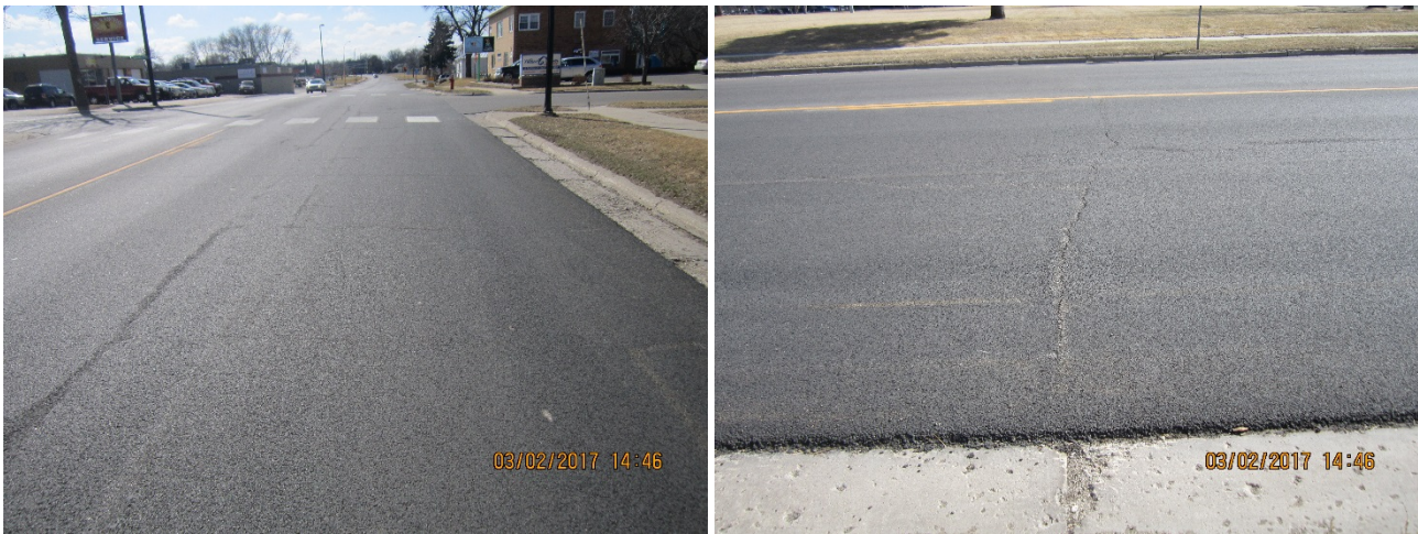
Figure 6 Minnesota Trunk Highway 19, 2017 performance of UTBWC mill and overaly in Marshall, MN
