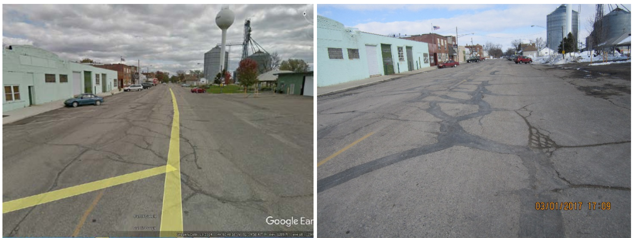
Figure 1 (Left) County Road 3 in 2014, prior to mastic. (Right) In 2017, after mastic.
