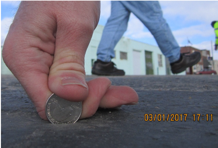
Figure 2 "Coin test" of mastic repair.
