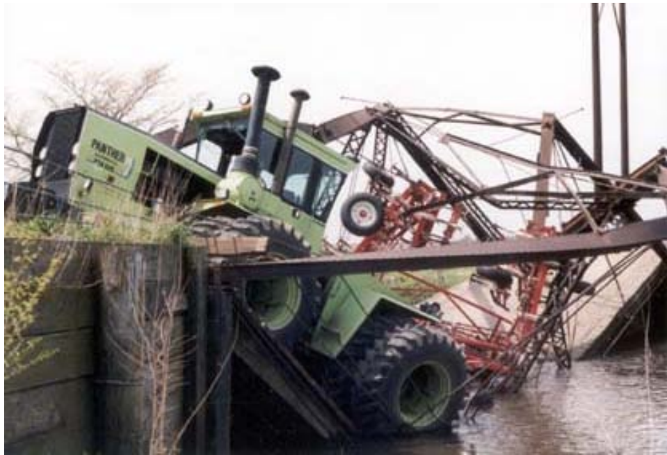
a. Bridge Number 1
