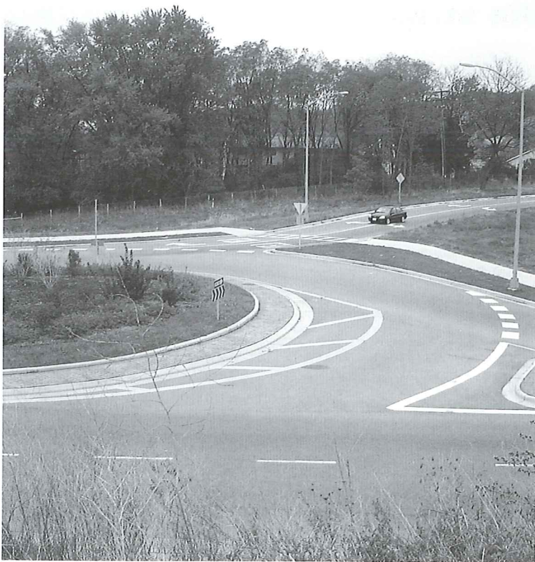
Converting a signalized intersection to a roundabout helps slow traffic, reduce conflict and improve safety.
