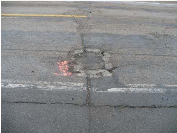
Figure 2 - Pothole filled using microwave and RAP 3-20-2009.
