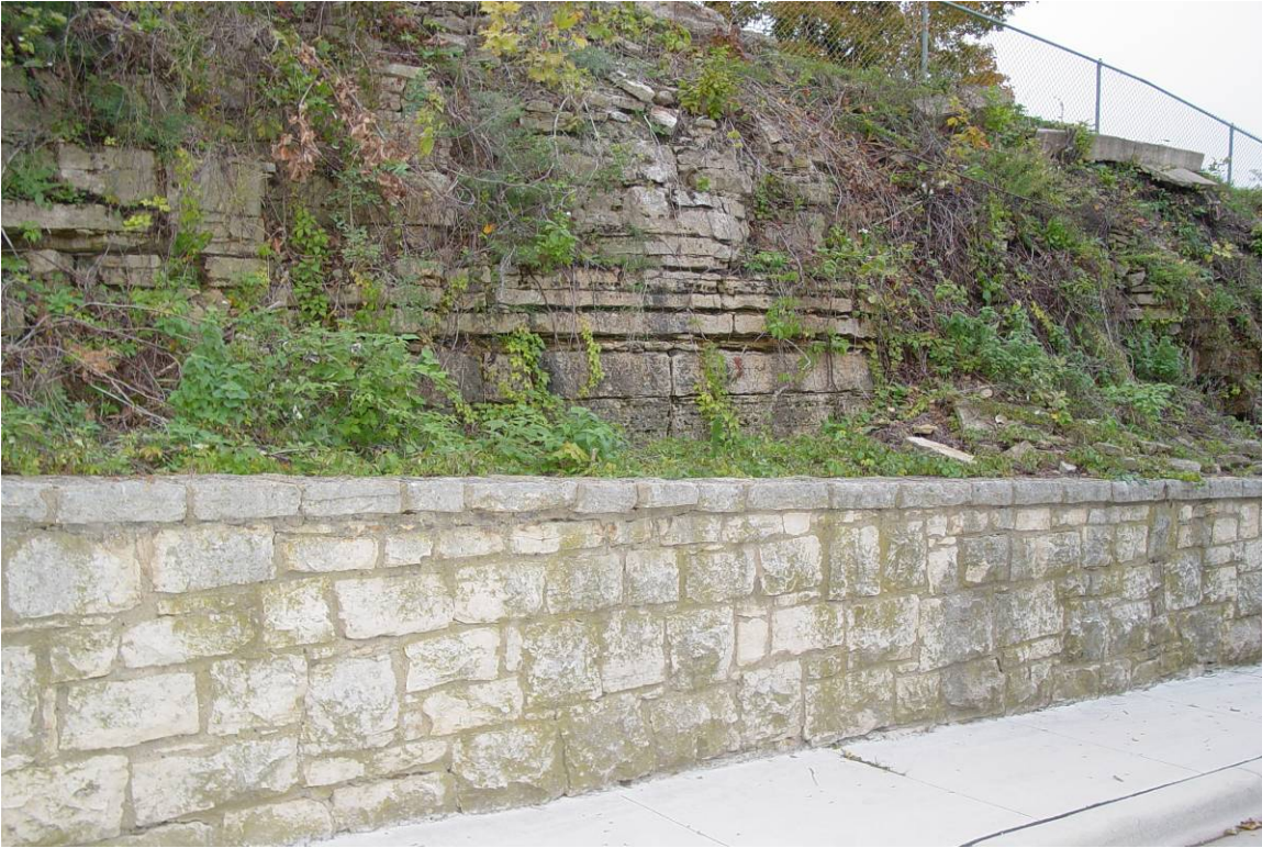
Plate 3. East retaining wall, showing typical orientation to limestone exposure, facing southeast
