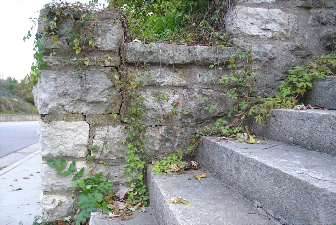
Plate 12. West retaining wall, north steps, facing south
