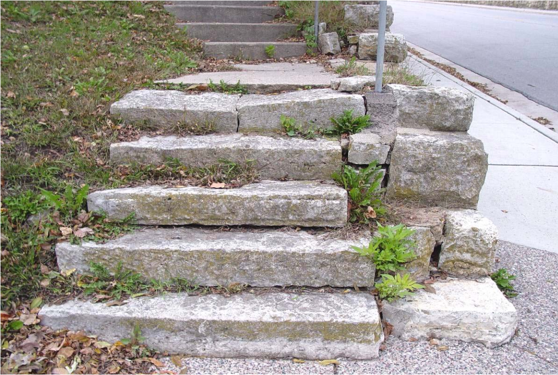
Plate 14. Masonry steps adjacent to west retaining wall, south end, facing north
