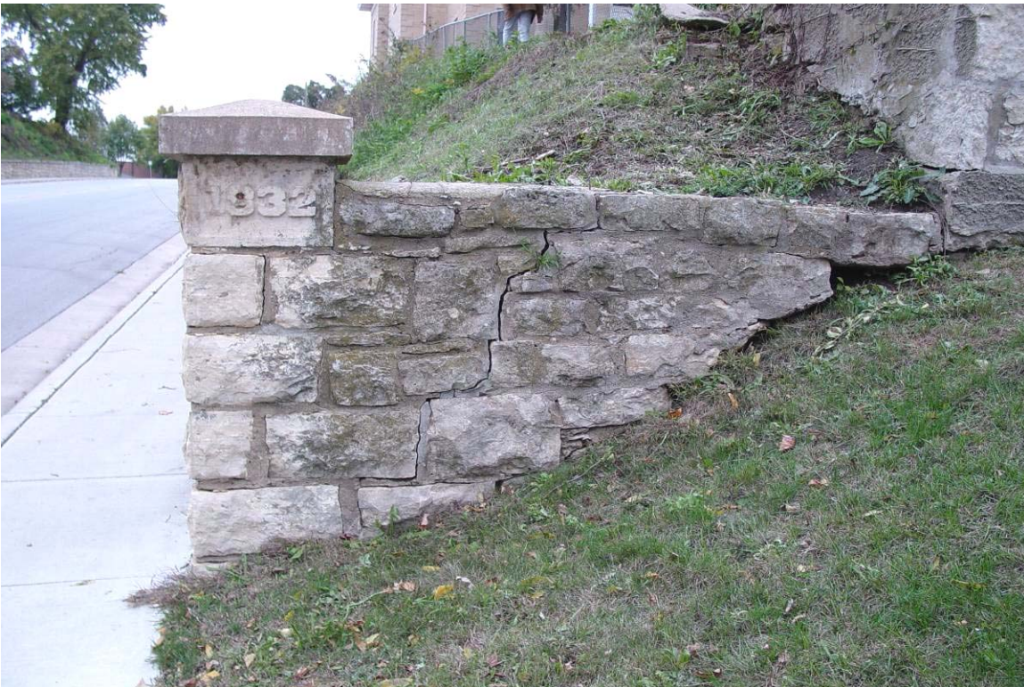
Plate 9. East retaining wall, south end, facing north
