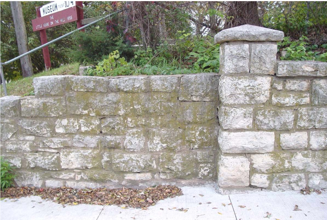
Plate 13. West retaining wall, south end, facing west
