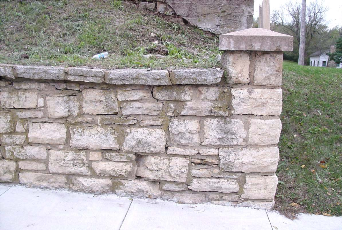
Plate 8. East retaining wall, south end, facing east
