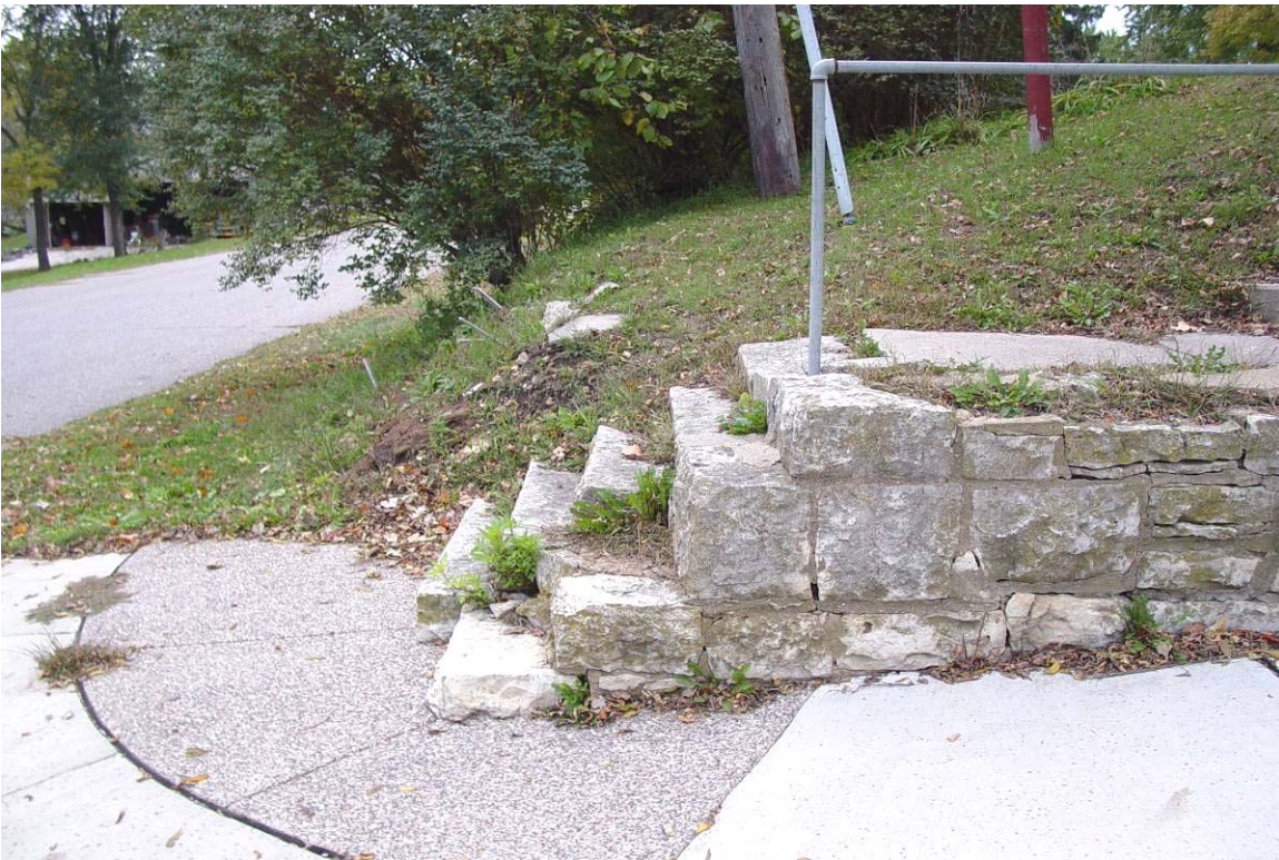
Plate 15. Masonry steps adjacent to west retaining wall, south end, facing west
