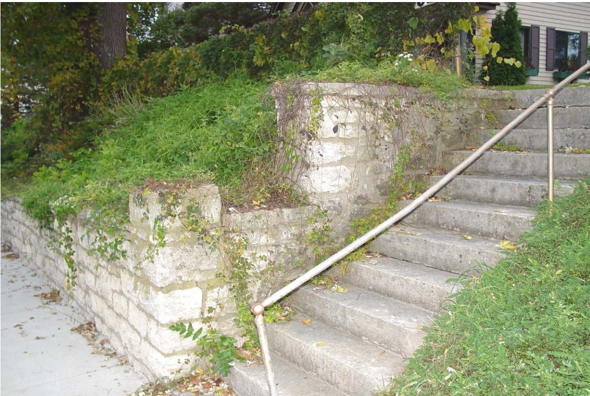
Plate 11. West retaining wall, north stone steps, facing southwest
