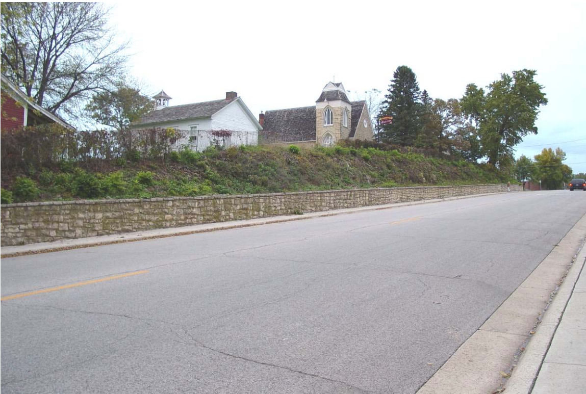
Plate 2. West retaining wall and adjacent historic properties, facing northwest
