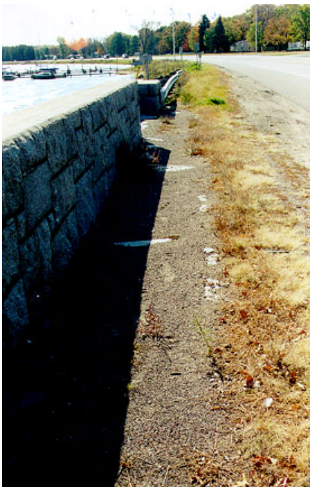
5. North Wall looking South ( Curb is not visible )
