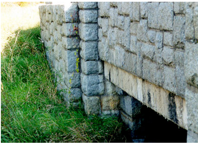
17. Culvert Opening (Note: Condition of granite header and surrounding mortar joints)
