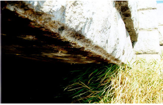
8. Close-up of Granite Header over Culvert
