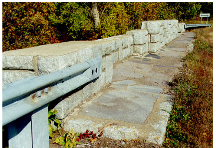
4. West Wall looking North
