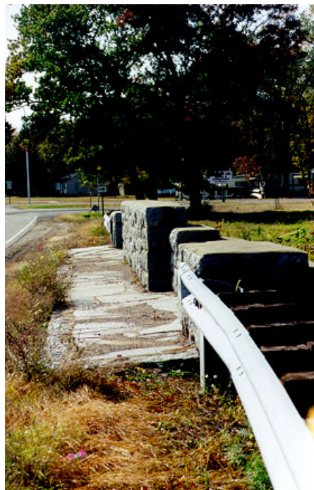
6. West Wall looking South ( overgrown turf )
