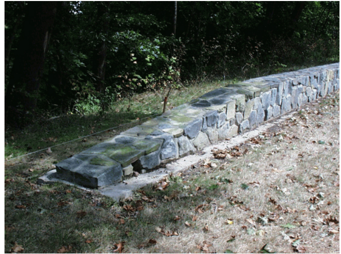
Stone Masonry Guardwall
